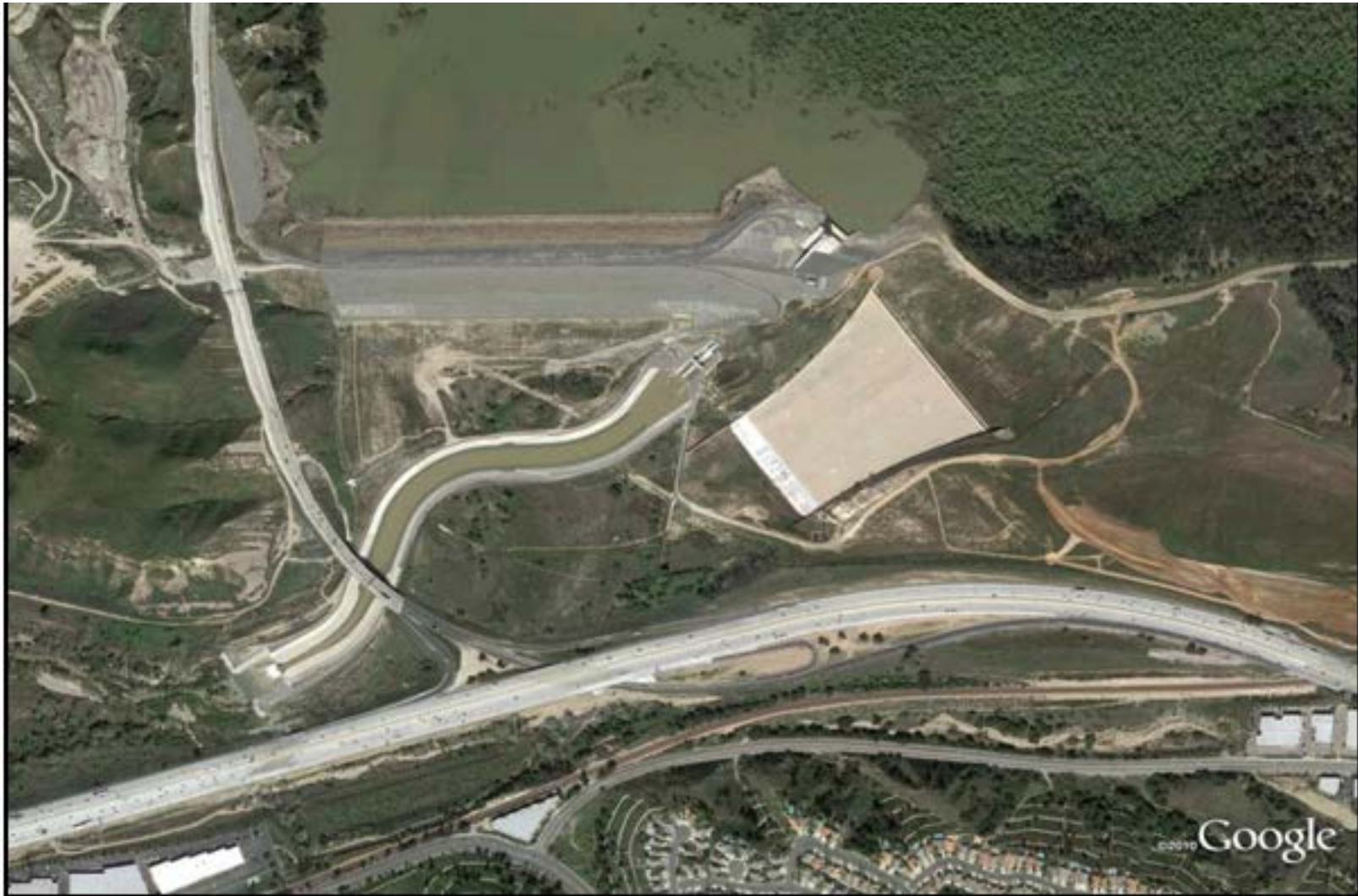
PRADO DAM & SPILLWAY, Corona, CA Originally Completed in May 1941 New Outlet Works and Dam Raise 2008
