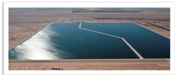
Warren H. Brock Reservoir, a System Efficiency ICS project funded by the Central Arizona Water Conservation District, the Metropolitan Water District of Southern California, and the Southern Nevada Water Authority.
