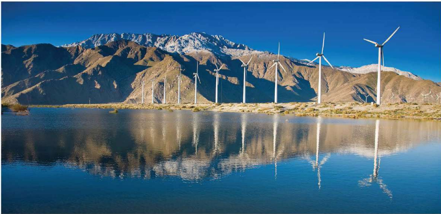
Coachella Valley Water District (CVWD) and Desert Water Agency (DWA) became State Water Contractors to supplement the natural groundwater replenishment from snow melt and rainfall with imported water. Since the imported supply first arrived in 1973, more than 2.8 million acre-feet of water has been replenished at the facility. Combined, CVWD and DWA have the third largest entitlement to State Water Project water at 194,100 acre-feet annually. There is no physical connection from state facilities to the Coachella Valley, so the two agencies trade with Metropolitan Water District of Southern California (MWD) for an equal amount of Colorado River water released from the Colorado Aqueduct. MWD also can “bank” water in the aquifer during wet years and get back an equivalent amount during dry seasons.
