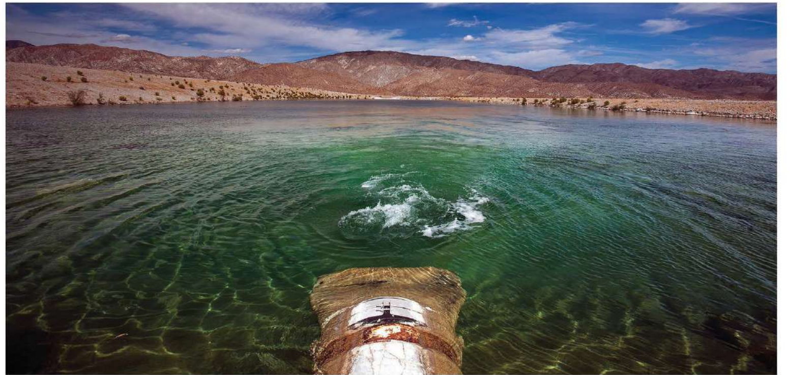
Replenishment at the Mission Creek Groundwater Replenishment Facility began in 2002 as a joint effort between CVWD and DWA. The agencies divert a portion of their State Water Project entitlement to the facility near Desert Hot Springs. To date, more than 143,438 acre-feet of water has been replenished at the site. Although the aquifer exists beneath the entire valley, subbasins restrict distribution of replenishment water so facilities are built where they will do the most good in reversing aquifer overdraft and ensuring reliable water supplies are available throughout the region. Groundwater replenishment is an important tool in reducing overdraft of the aquifer and a key component to CVWD and DWA’s long-term groundwater management plans.
