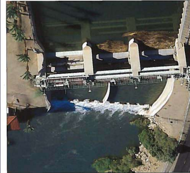
IMPERIAL DAM, above, raises the Colorado River 25 feet and diverts water into the All-American and Gila Gravity Main canals. Much of the sediment that could clog the canals is removed here at the desilting works near Yuma.
