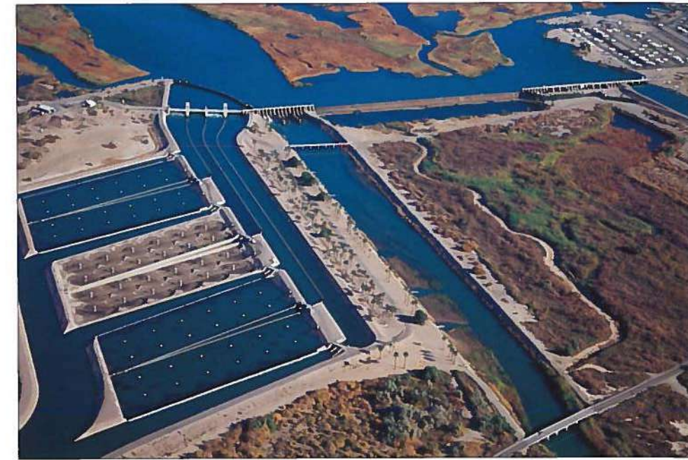
IMPERIAL DAM, above, raises the Colorado River 25 feet and diverts water into the All-American and Gila Gravity Main canals. Much of the sediment that could clog the canals is removed here at the desilting works near Yuma.
