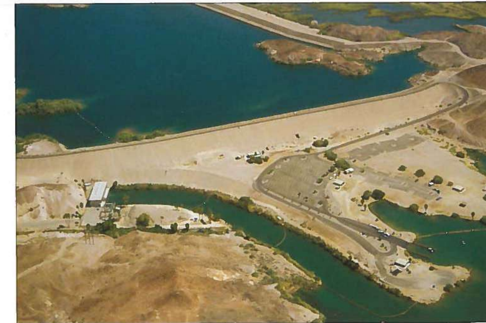
SENATOR WASH DAM, right, and its reservoir are used to improve water delivery scheduling. Colorado River water released from Hoover Dam but not immediately needed is stored here until it is needed, then released.
