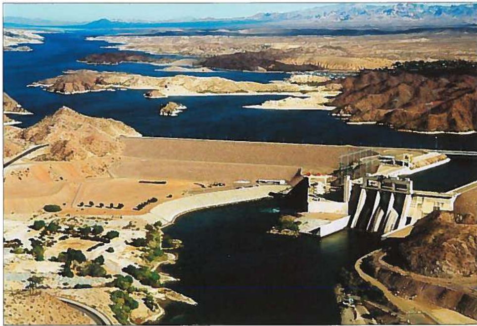
DAVIS DAM, above, is 67 miles downstream from Hoover Dam, 88 miles upstream from Parker Dam. The Mexican Treaty of 1944 required the United States to build the dam for regulation of water delivered south of the border.
