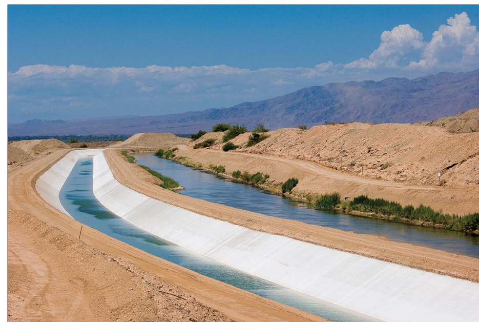
The newly lined section of canal was built parallel to the unlined version to avoid a disruption of service. The unlined section was taken out of use shortly after the lined version was completed.
