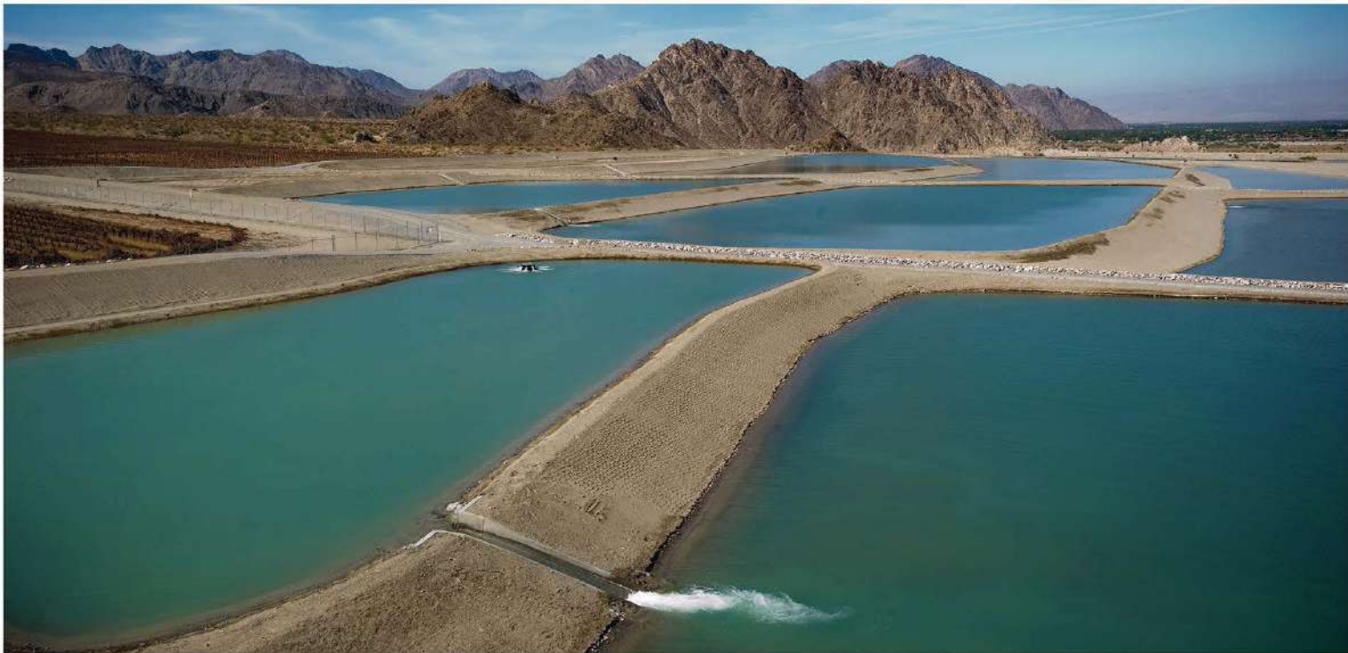
In 2009, CVWD’s Thomas E. Levy Groundwater Replenishment Facility in La Quinta became fully operational with the ability to replenish up to 40,000 acre-feet of water annually. The facility started as a pilot project in 1997. To date, more than 147,000 acre-feet of water has been replenished at this facility. Groundwater levels at many nearby wells have risen dramatically, showing the importance of the groundwater replenishment program in reducing overdraft of the aquifer. Replenishment is among many methods used to protect and preserve local groundwater supplies, including conservation and the use of Colorado River water or recycled water for irrigation, instead of groundwater.
